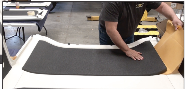
FIG. 15 & Fig 16 Slowly pull the release liner off as you press the piece into place. NOTE: Use gentle pressure. DO NOT use a lot of pressure when pressing piece into place.
