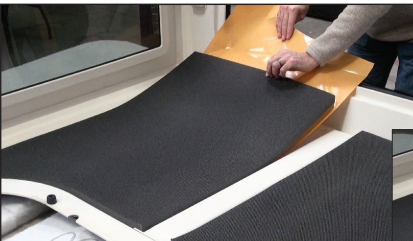
FIG. 11 & Fig 12 Slowly pull the release liner off as you press the piece into place. NOTE: Use gentle pressure. DO NOT use a lot of pressure when pressing piece into place.
